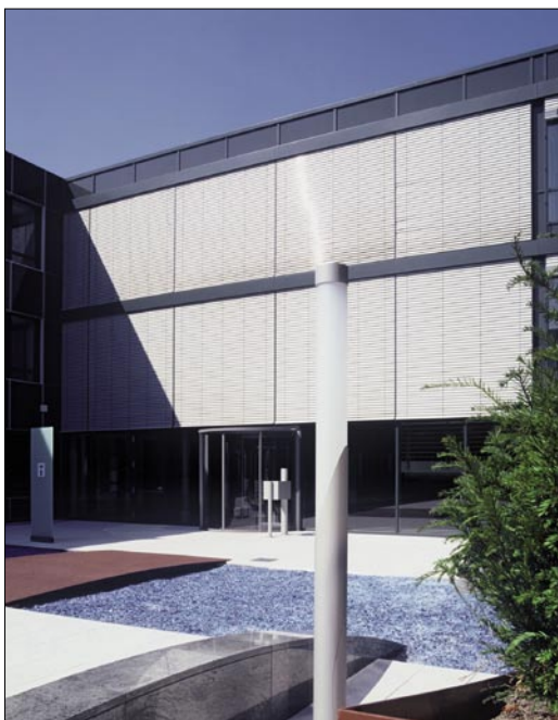
Büro Center / Office Center
